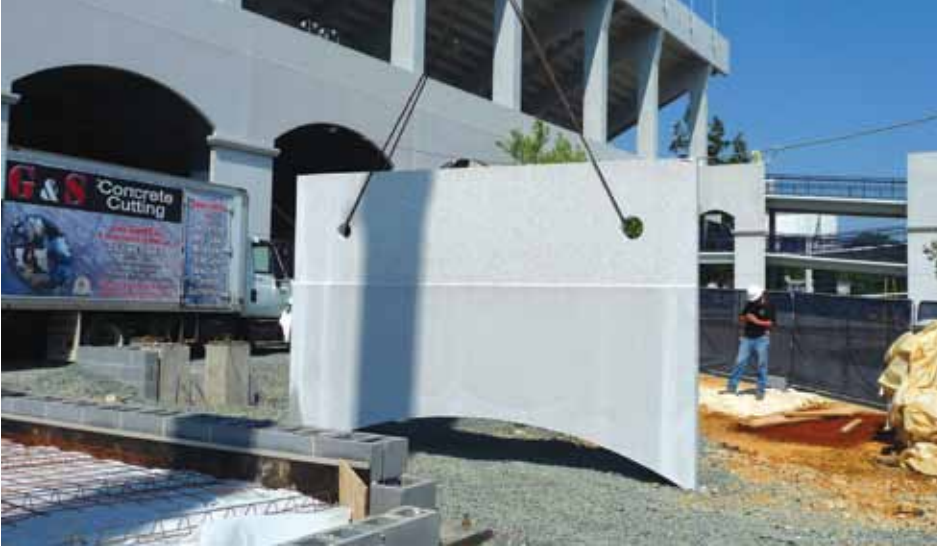
The 8-inch-thick concrete sections were lowered by crane.
